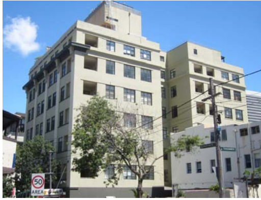
Figure 42 74-80 Reservoir Street was designed for retailer Murdoch's Limited in 1921 by Joseland & Gilling.
