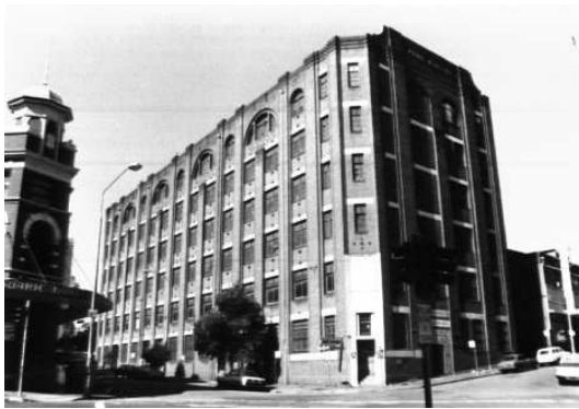
Figure 44 Mark Foy's Warehouse at 52-68 Commonwealth Street was designed by Spain Cosh & Dods in 1917.
