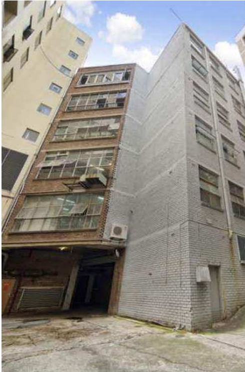
Figure 25 Rear of building – 1970s additions
