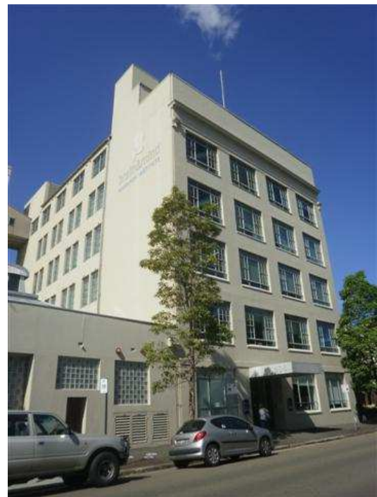
Figure 14 100-106 Mallett Street. Source: State Heritage Inventory.
